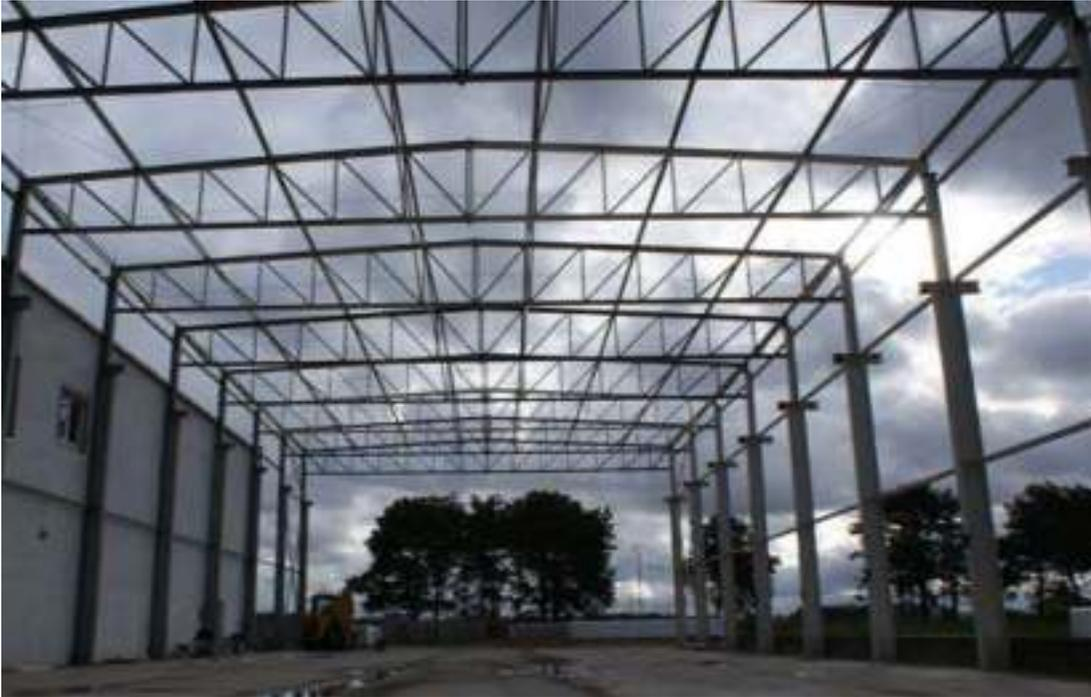
COMBINATION OF STEEL & RCC STRUCTURE
